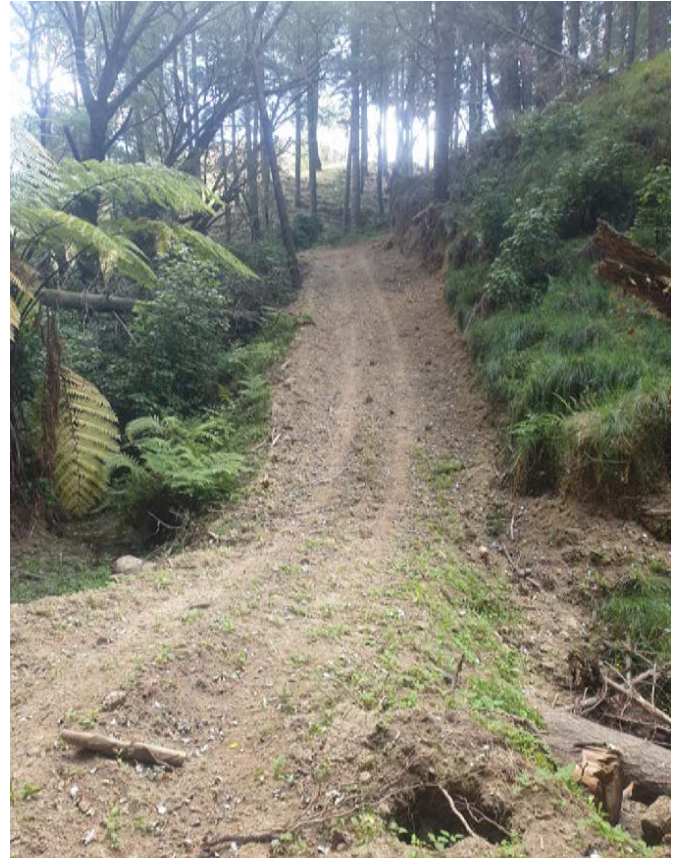
Track repaired in stand 1
