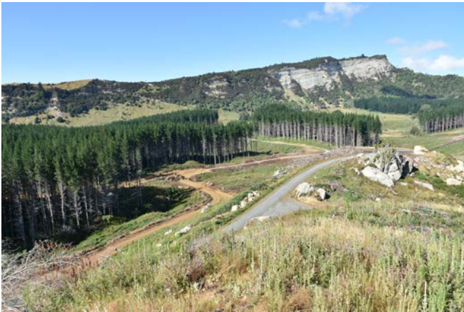
Overview of roads
