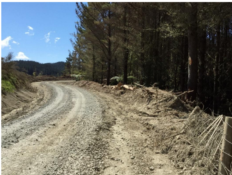
Pic 2: Roading work completed on Tarewa Road, Winderemere Forest to the right.
