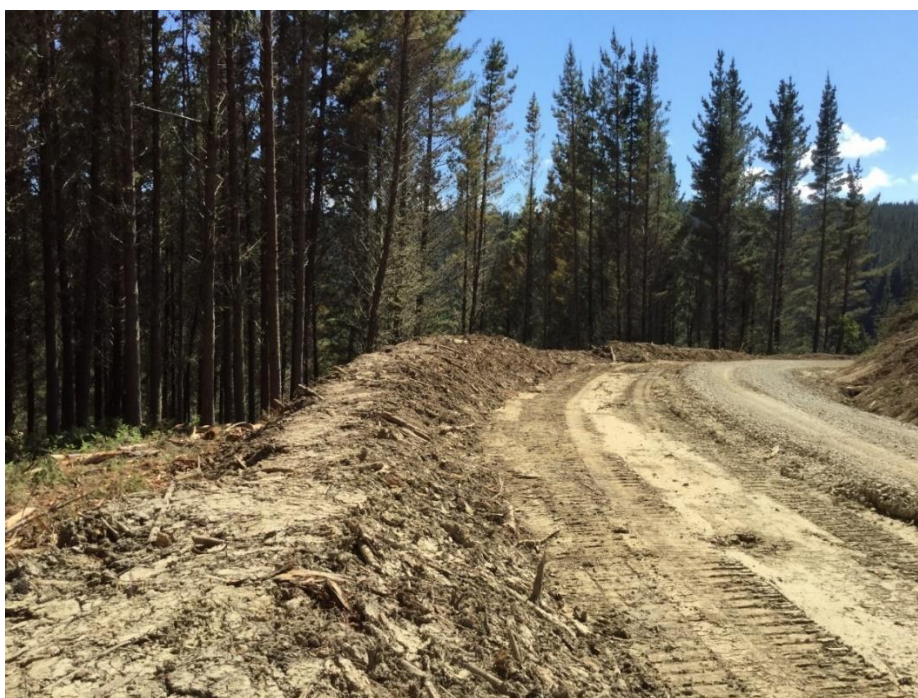
Pic 3: Roading work completed on Tarewa Road, Winderemere Forest to the left.
