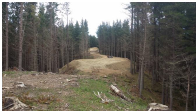
Roadline into Skid 10 – The Island
