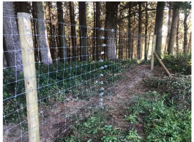
Boundary fence that required urgent attention is now repaired
