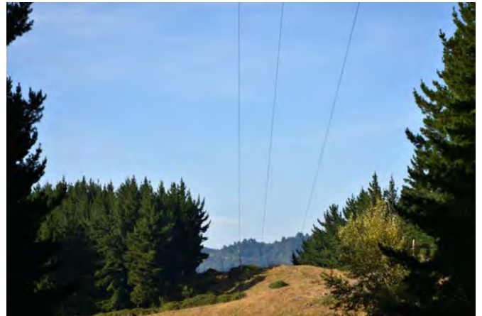
Powerline corridor clear
