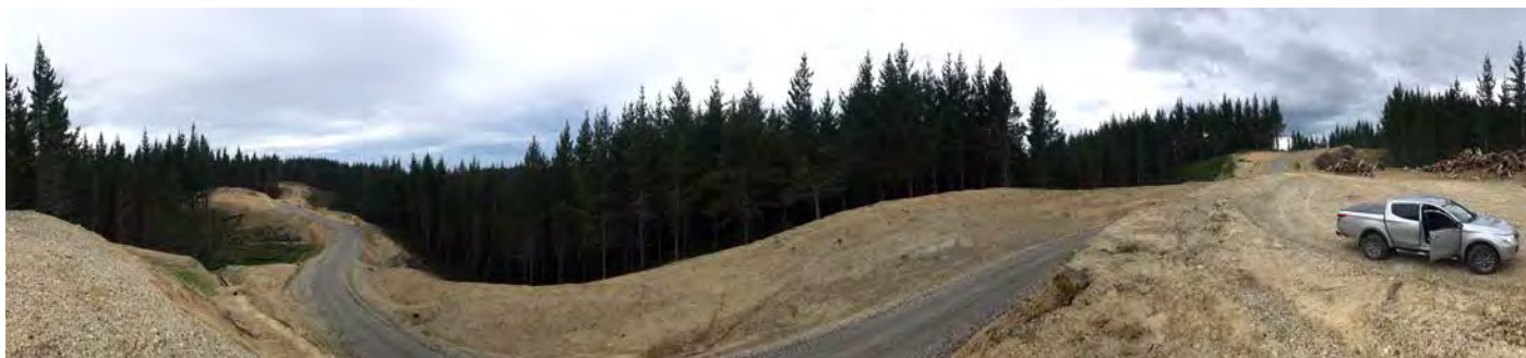
Overview of the forest road formation
