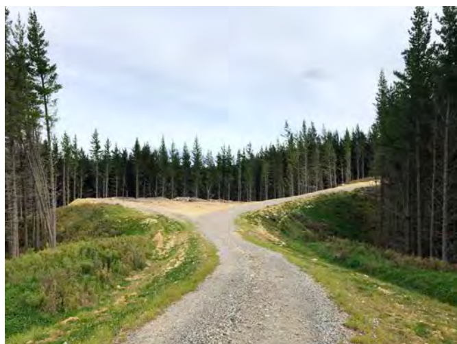
Forest roads are in very good condition
