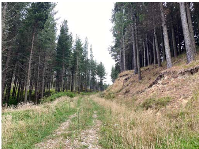
Road that requires maintenance
