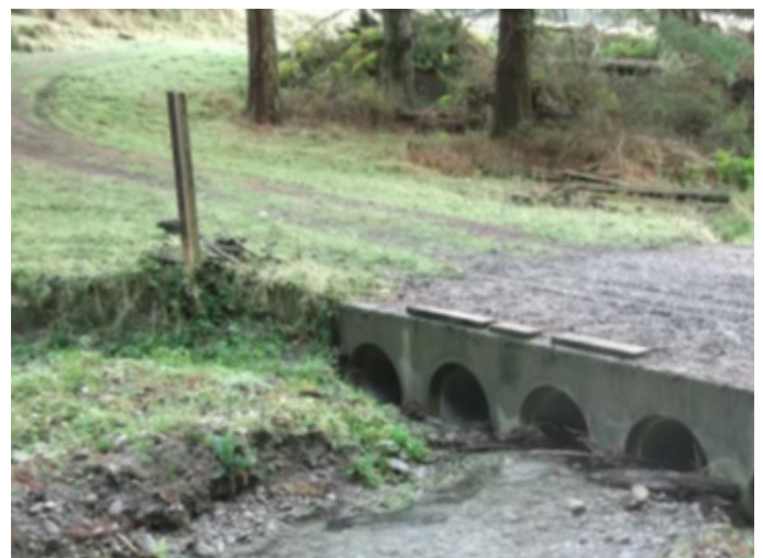
Culvert crossing at the main entrance
