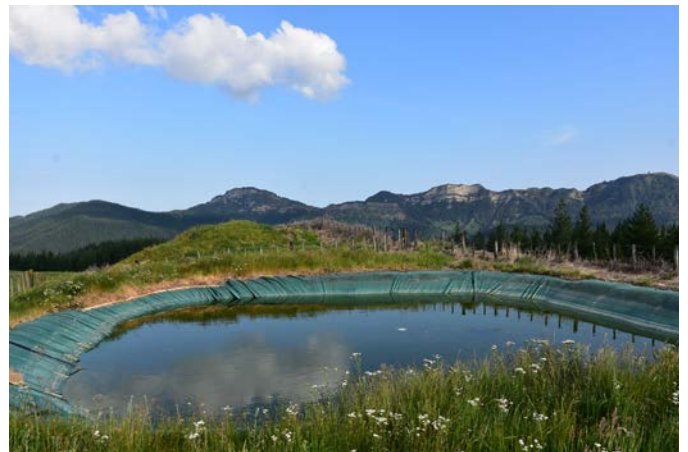
Fire pond on airstrip in good condition
