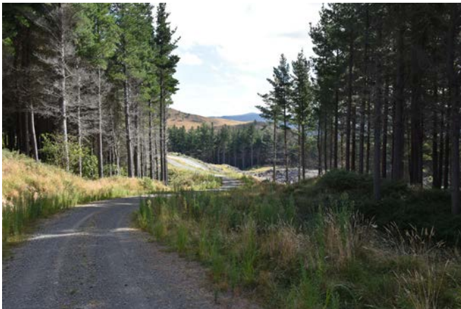
Forest roads are in good condition
