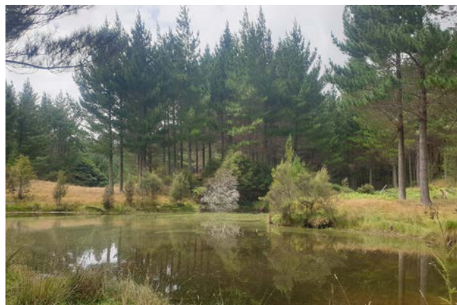
Dam has reasonable water level
