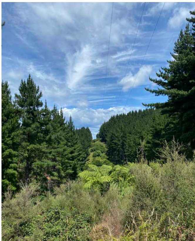
Power line corridor
