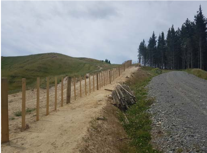
New boundary fence
