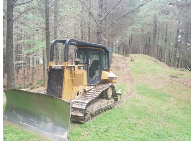
Digger for tracking work in December
