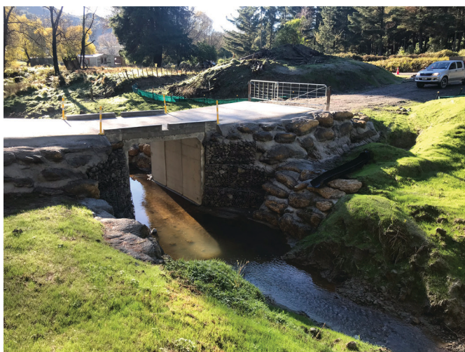
New entrance prior to sealing
