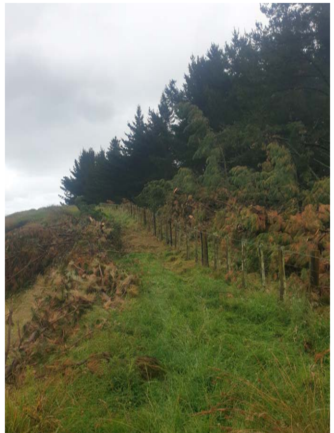
Boundary fence repairs
