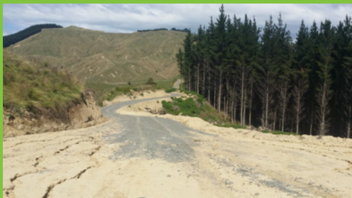
Road into the top skid
