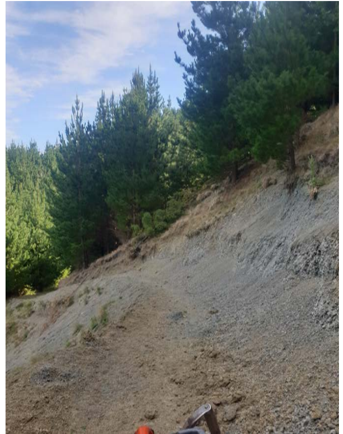
Section of repaired track in stand 10
