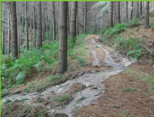
Track scouring following heavy rainfall
