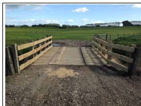
The bridge at the run-off after it had been repaired.
