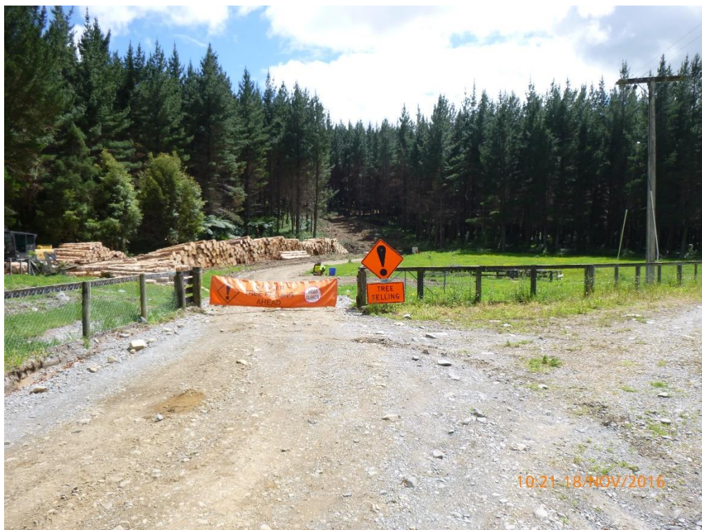
Commencement of road line salvage at the complex.
