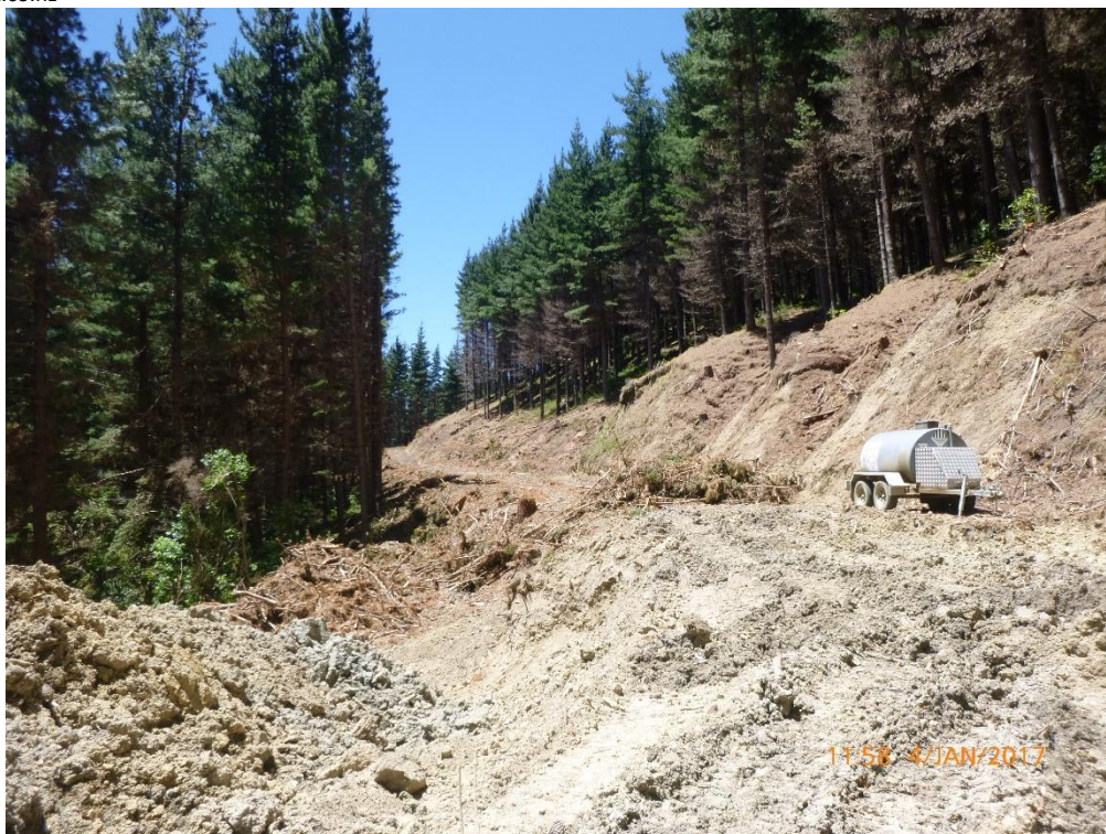
Image 3. Road line salvage from crossing back towards Cricklewood - Woodlands boundary.
