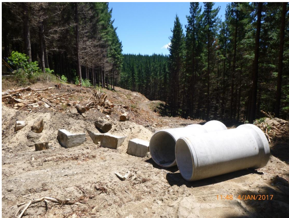
Image 1. Road line salvage commencing at Cricklewood Forest boundary
