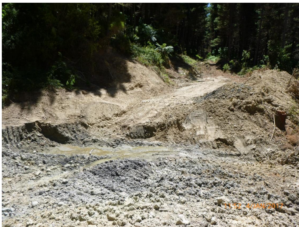
Image 2. Culverted crossing with boiler carcass removed.
