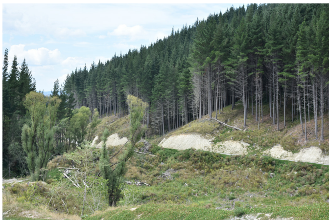
Roads are in good condition
