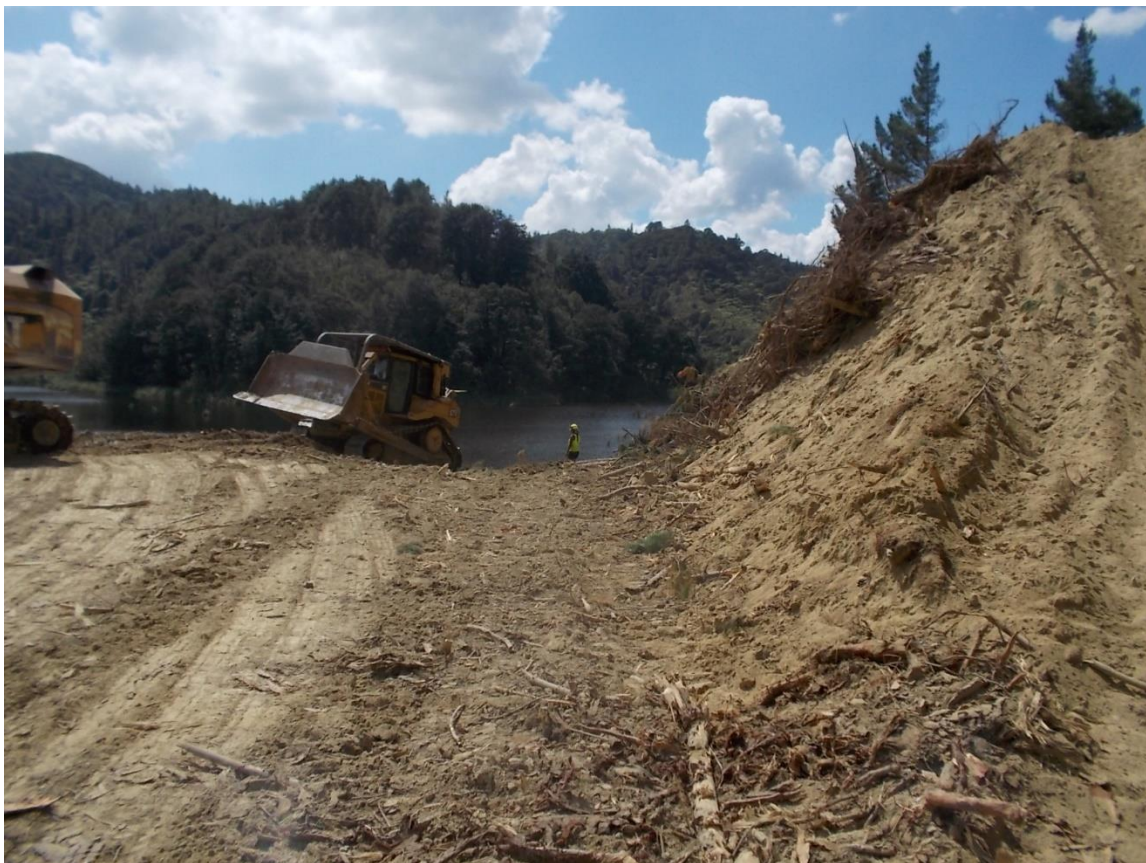
Figure 2: The Dozer bringing out another drag to landing 26 on Reid Road.
