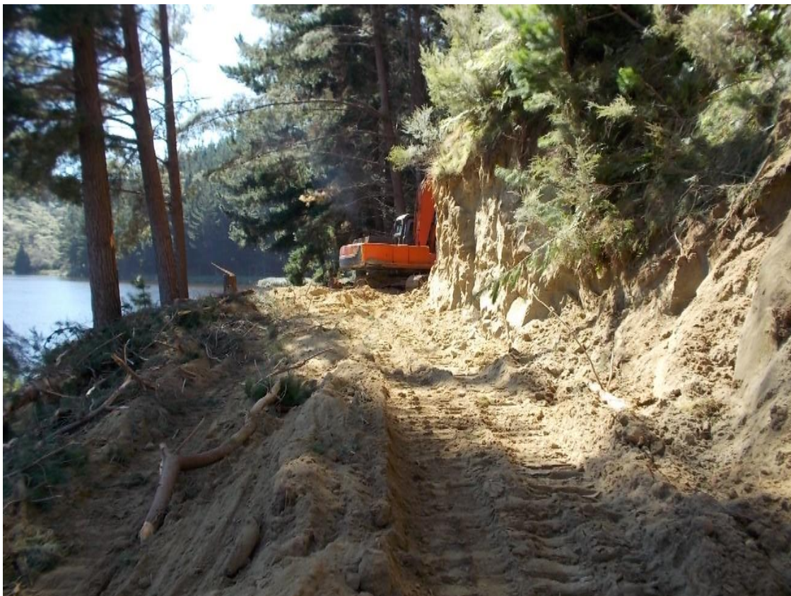
Figure 5: The ground base crew widening the track around Lake Waikare.
