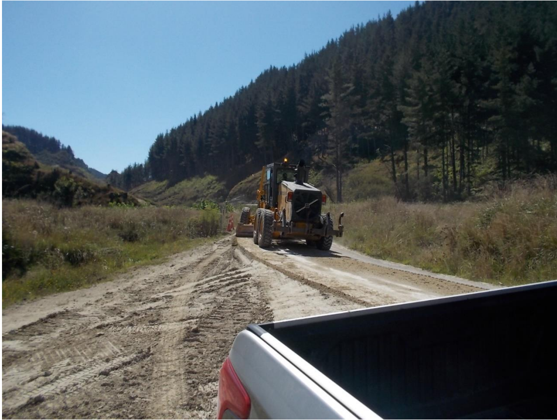
Figure 4: Waikare Road in the process of being graded.
