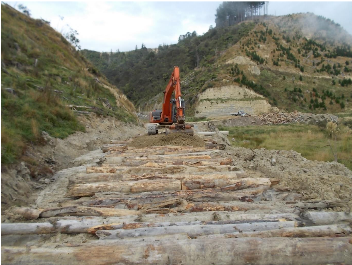
Figure 3: Laying Corduroy and metal on Hope road.
