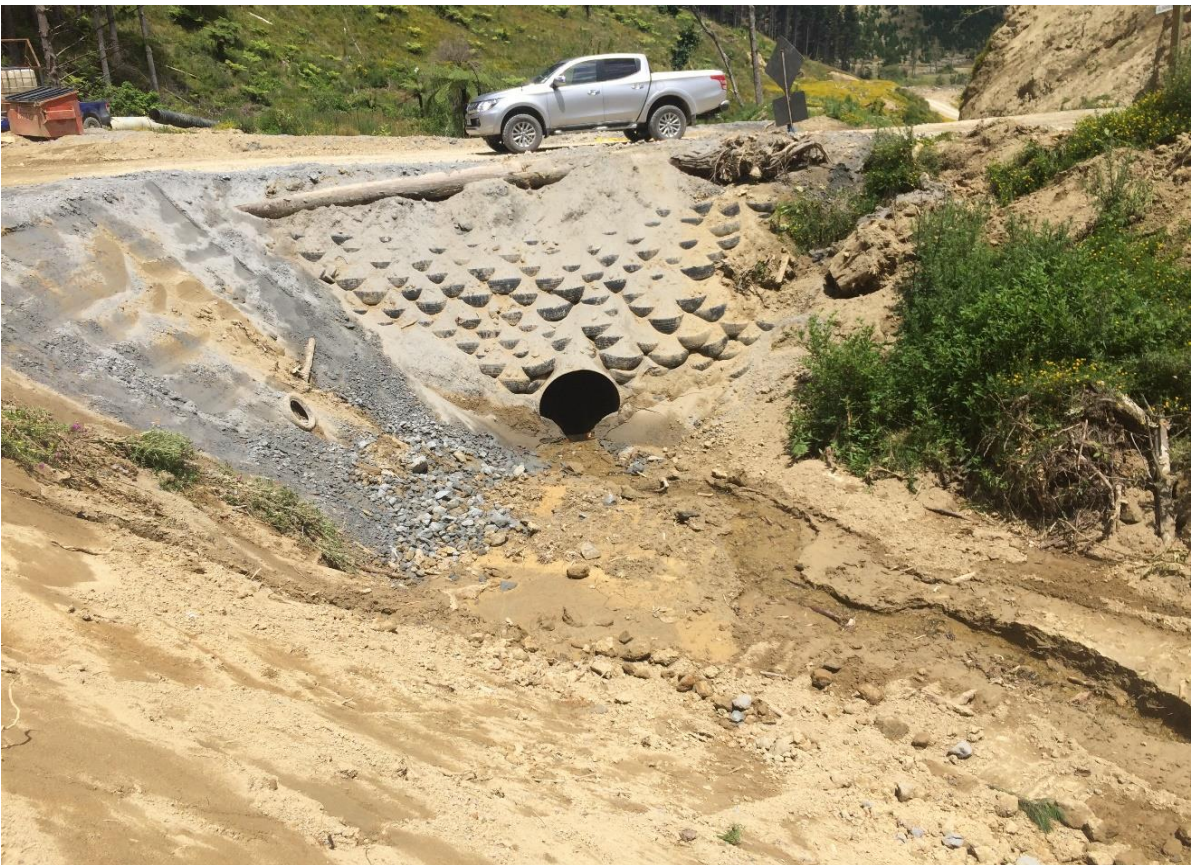
Figure 5: The finished job, note the tire head wall.
