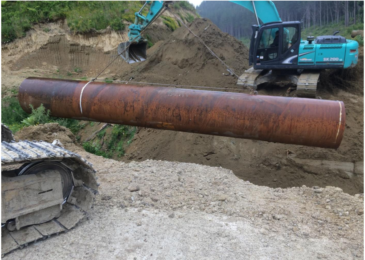
Figure 4: A section of culvert pipe being lowered into the culvert at the Gardner Gillingham Road intersection. This repair was carried out over the Xmas break to avoid disruption to the harvest crew.
