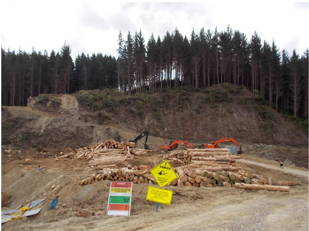
Figure 3: Hughes Rd landing 30, the ground based crew spent the whole month pulling to this skid site.
