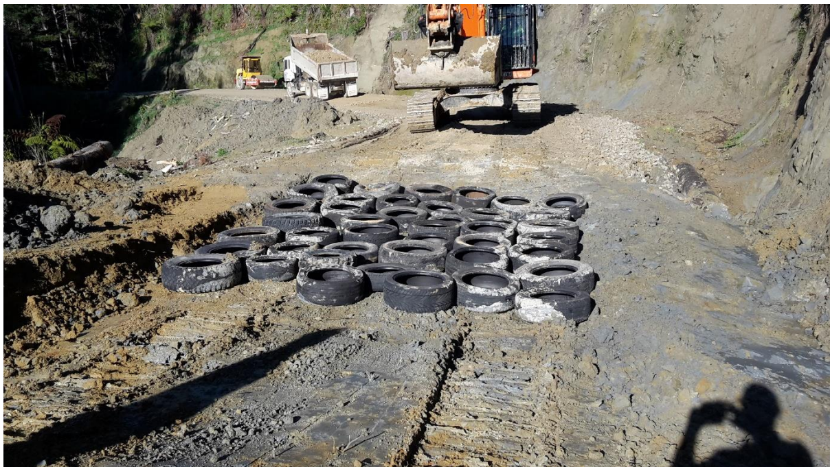
Figure 2: Cellular confinement trial – using old tyres (See appendix 3).
