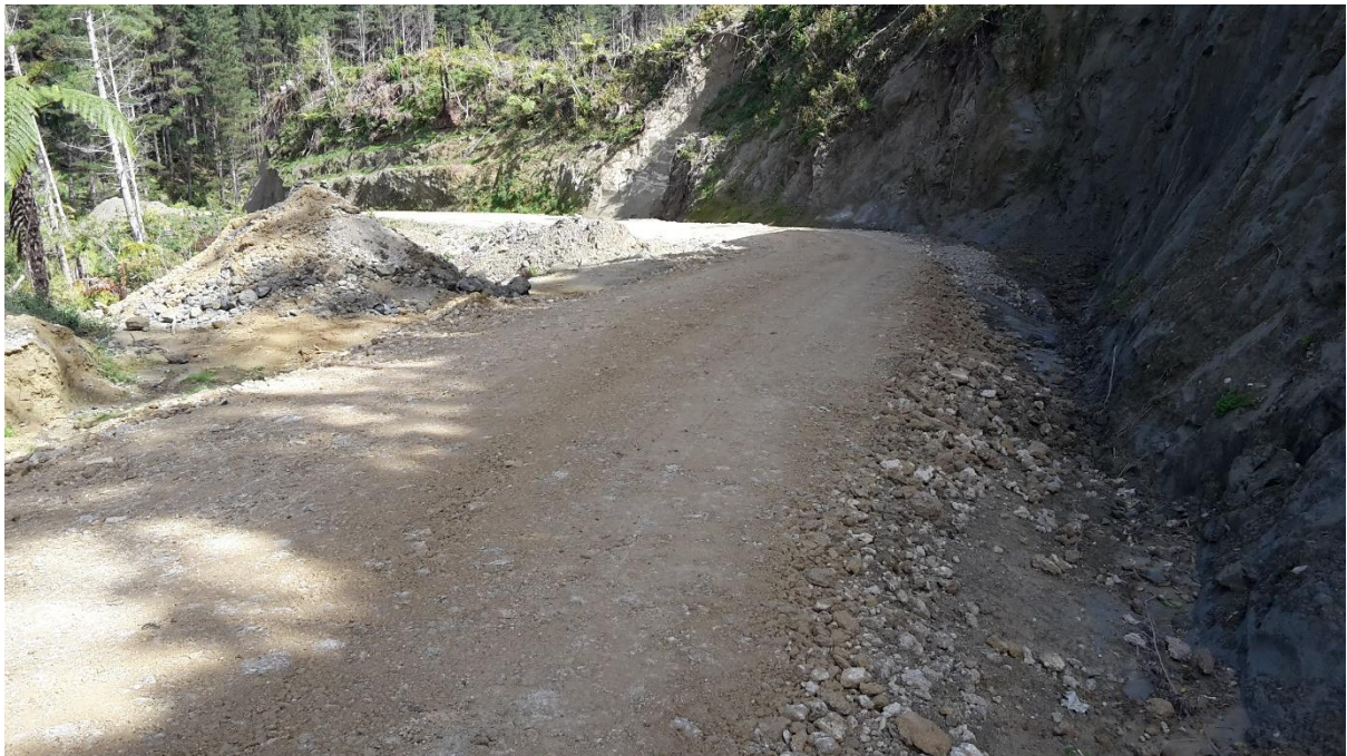
Figure 5: Tyre trial - after repair
