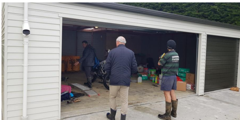
Photo: Roger Dickie, Jack Ballam and Ben inspecting finished garage
