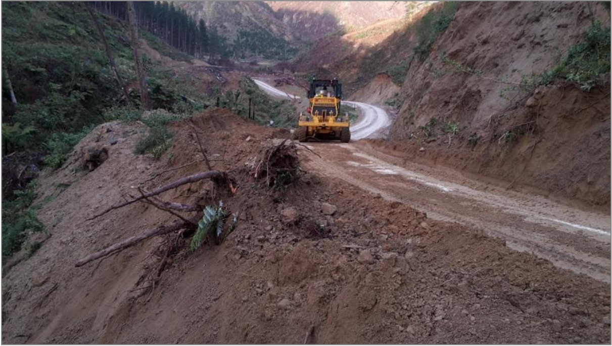
Figure 2: Maintenance clearing slips – Gillingham Drive.
