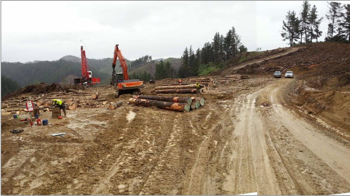
Figure 1: Log landing 40, end of Dickie Drive
