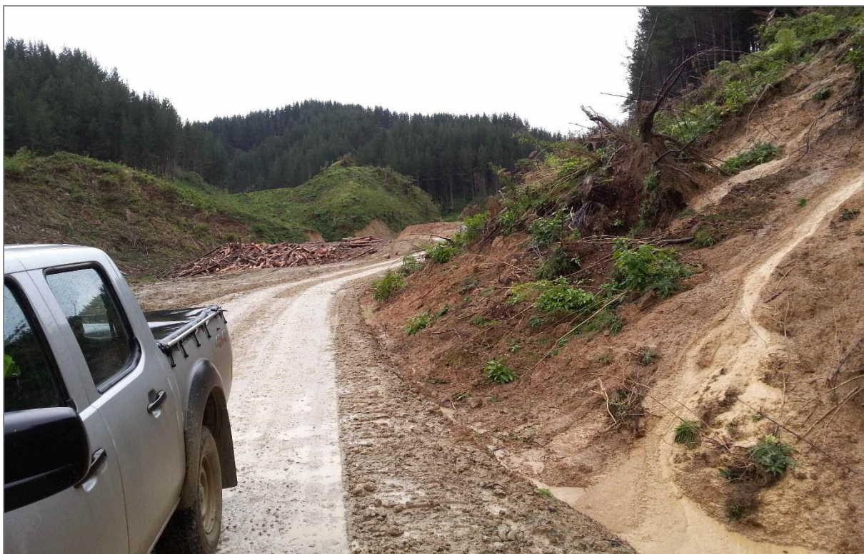
Figure 5: Slips blocking the watertable on Gillingham Road.
