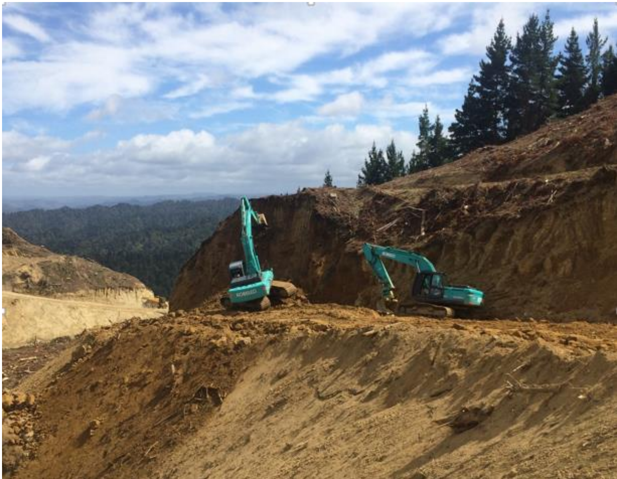
Figure 2: Grantson's Road in the process of being constructed.
