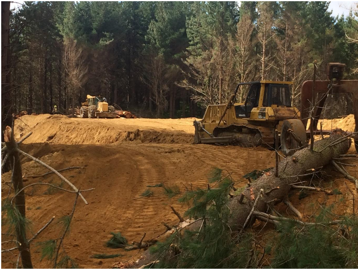
Figure 3: Skid 24 as first few logs are being pulled onto it.
