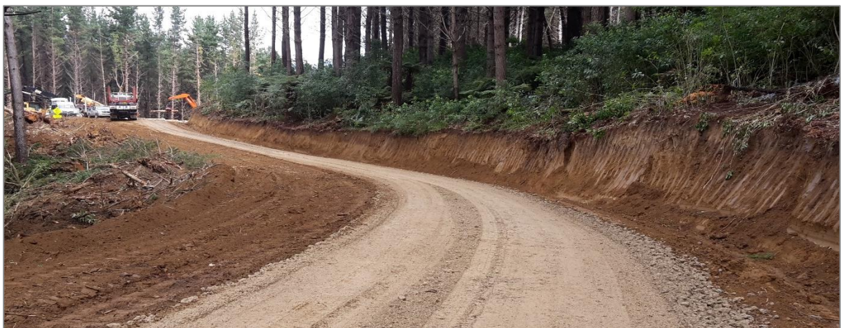
Figure 2: New construction on Dickie Drive.
