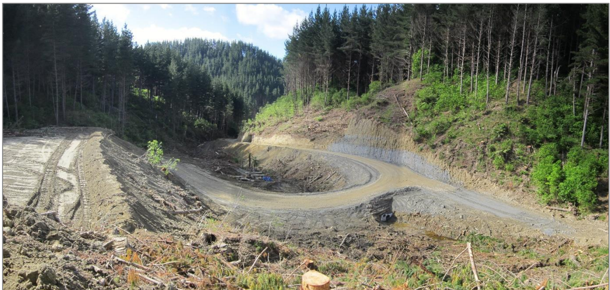
Figure 1: Culvert installation & landing 47 – Gardiner Drive
