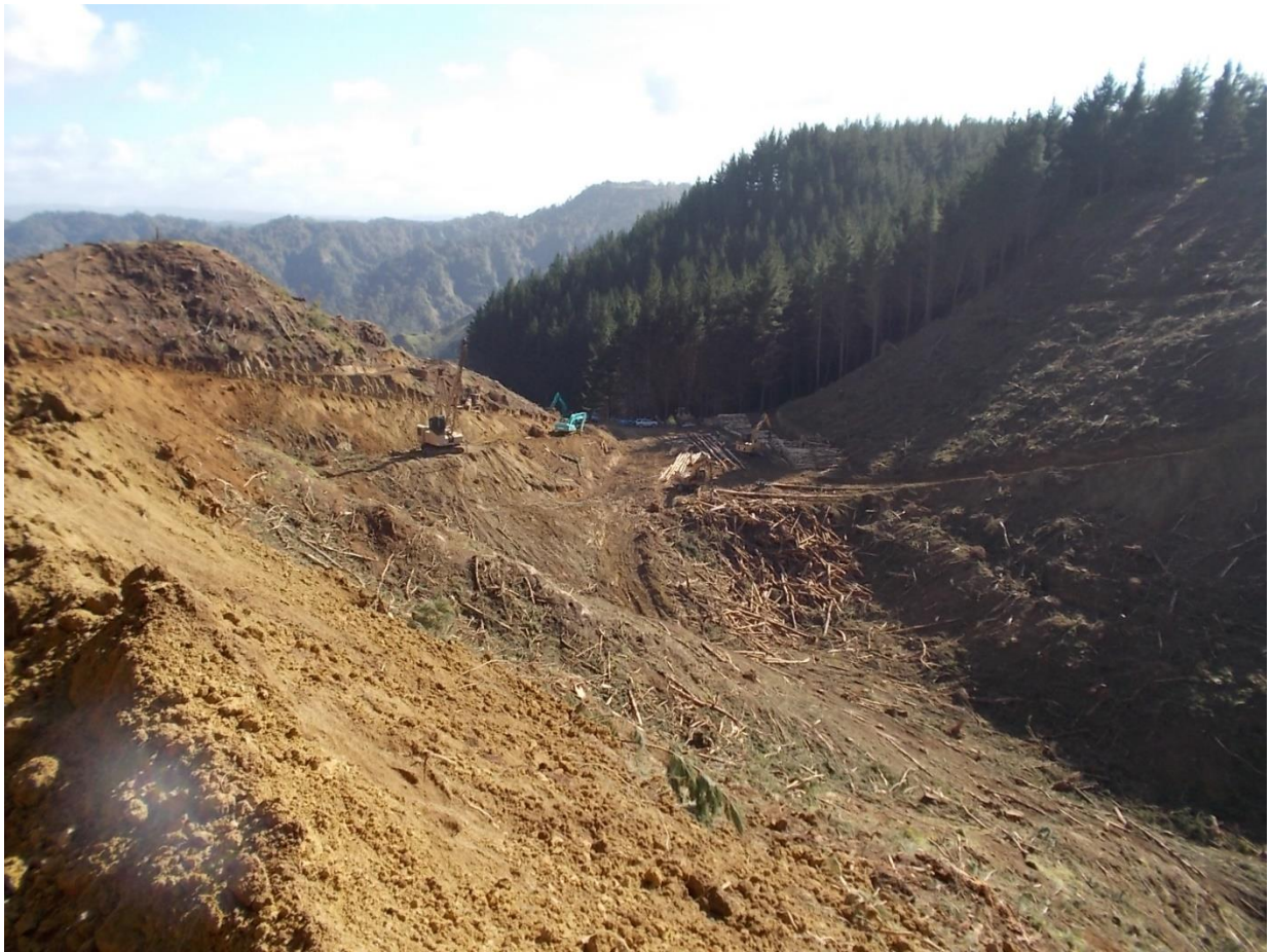
Figure 5: Skid 6 - the harvesting contractor and roading contractor (Blue Excavators) working together to open up the forest. Figure 4 on the previous page shows this face prior to the Hauler pad being established and was taken from the opposite face.
