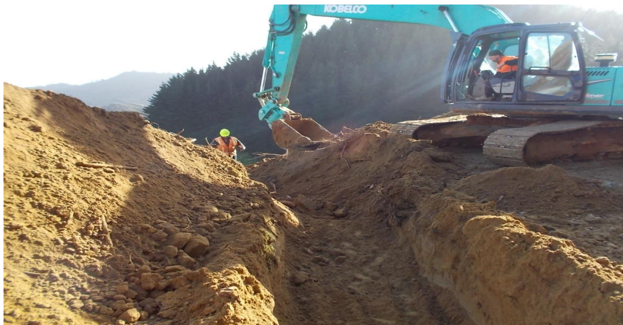
Figure 2 Culvert installation on CNL Road.
