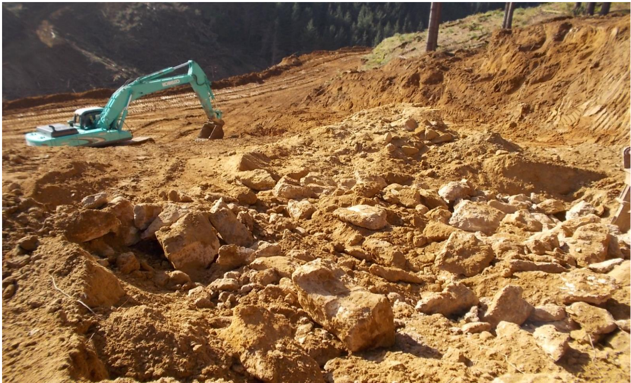
Figure 1: Shell rock being extracted from the Borrow pit on Selderbeek Road
