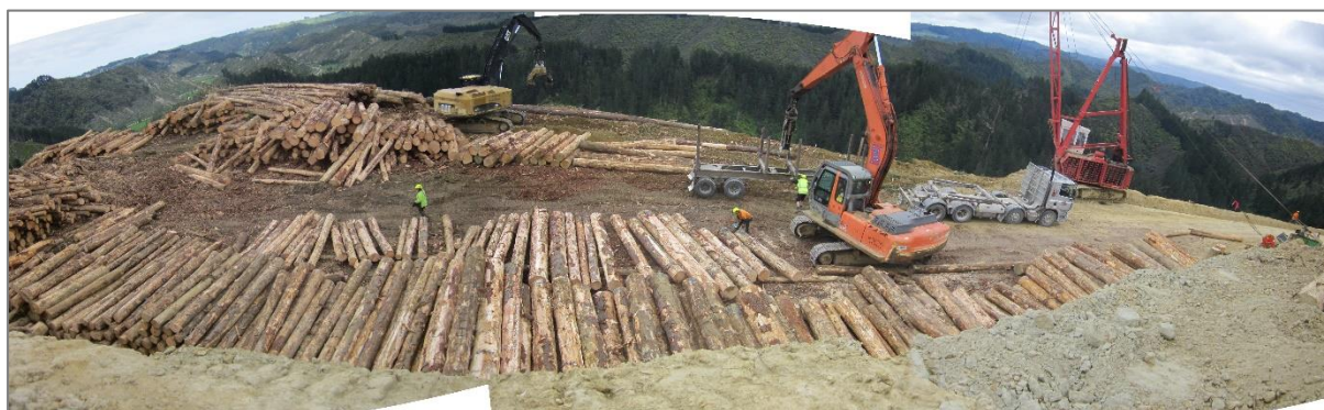
Figure 1: Landing 9 nearing completion
