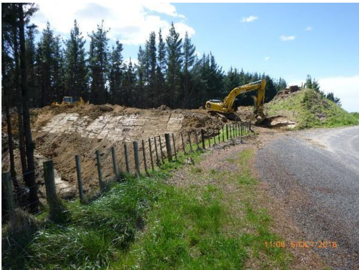
Figure 1: Setting 503 Temp Skid
