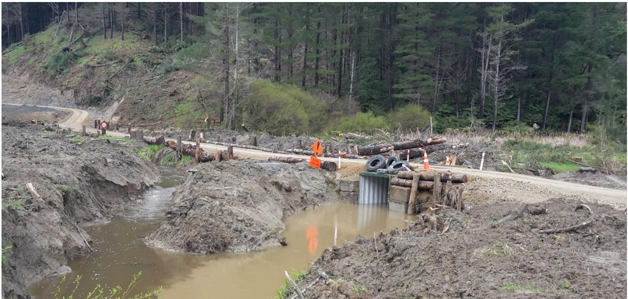
Figure 1: First culvert installation leading into compartment 2&3, Gillingham Road
