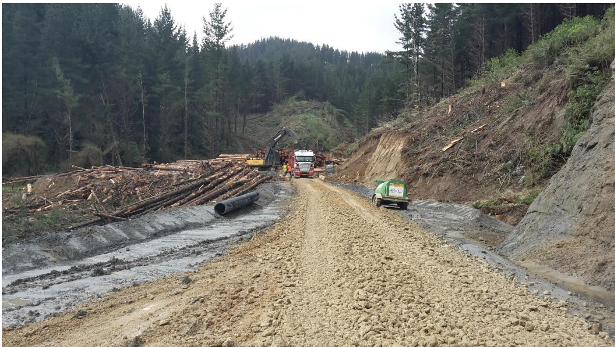
Figure 3: Roadlining continues into compartment 2&3.
