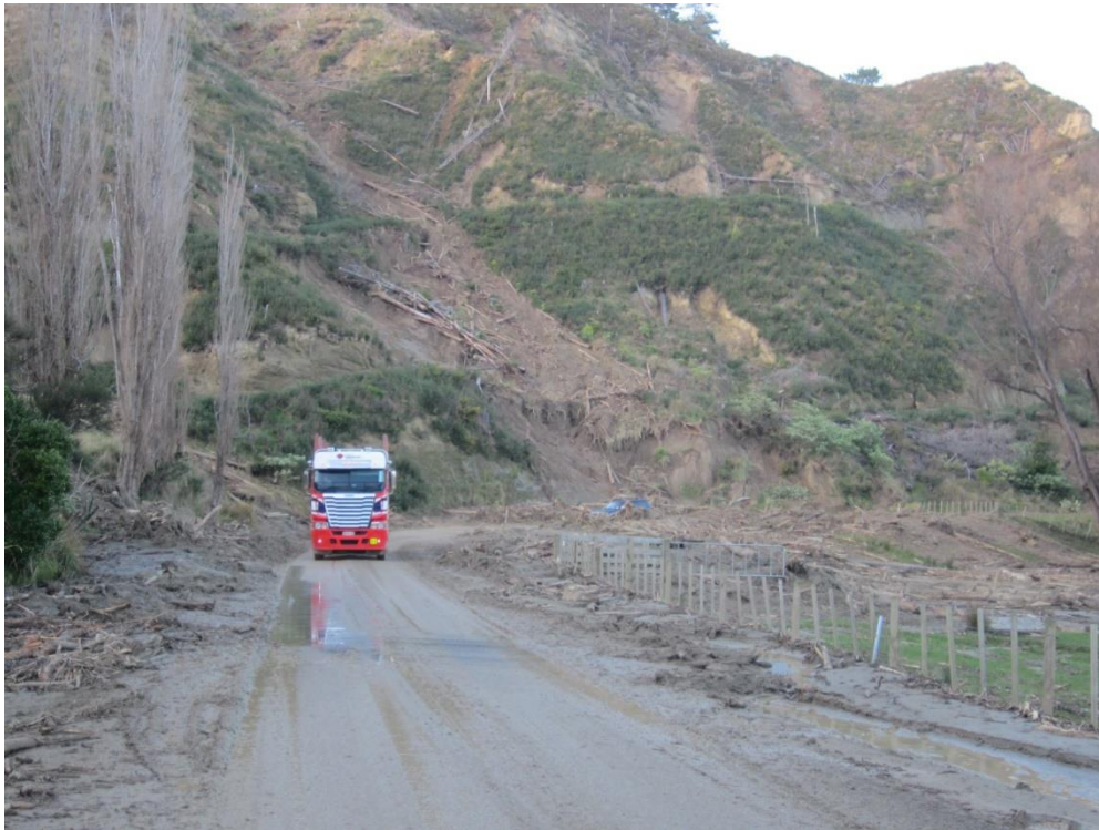
Figure 5 Cleared section of Waikare road
