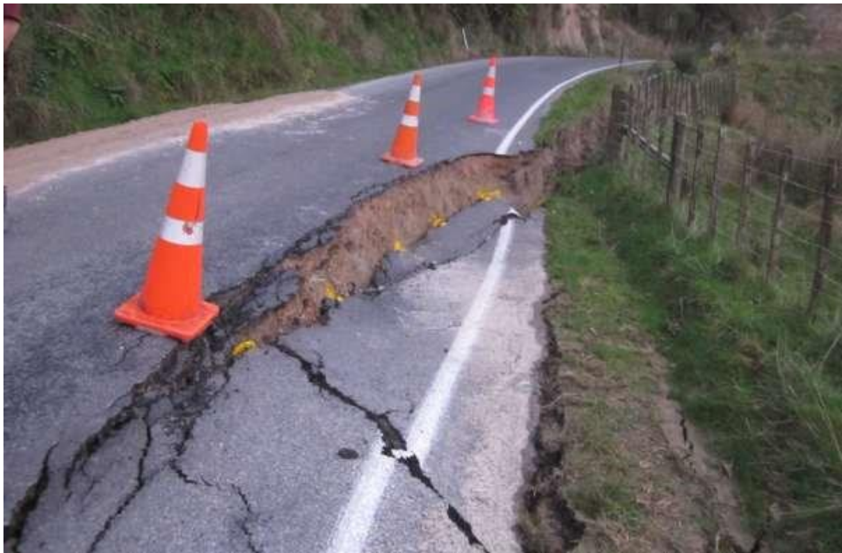
Figure 6 below shows the section of Mangawhio Road under repair.
